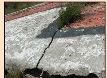
The upper arms of the “imperishable token” were removed, new concrete was placed, and the “I” visible today was established.
